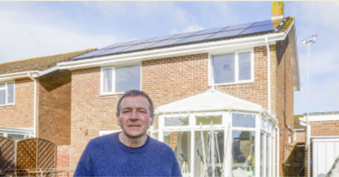
Ron, Salisbury 14 panels and battery storage installed
